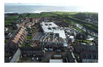
It is estimated around 5,000 tonnes of concrete will be used. Once poured and polished, the concrete will then take around four weeks to cure. During this time the groundworks around the structure will continue at pace and work will be done to fireproof the steel frame ahead of the external building material being installed.
